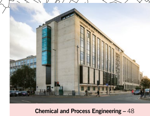
Chemical and Process Engineering – 48
